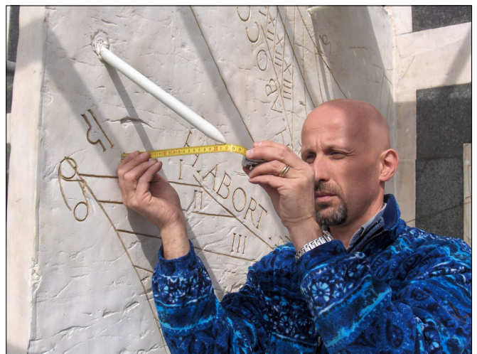
Fig. 7. Setting up the gnomon for the eastern Bohemian hours sundial.
